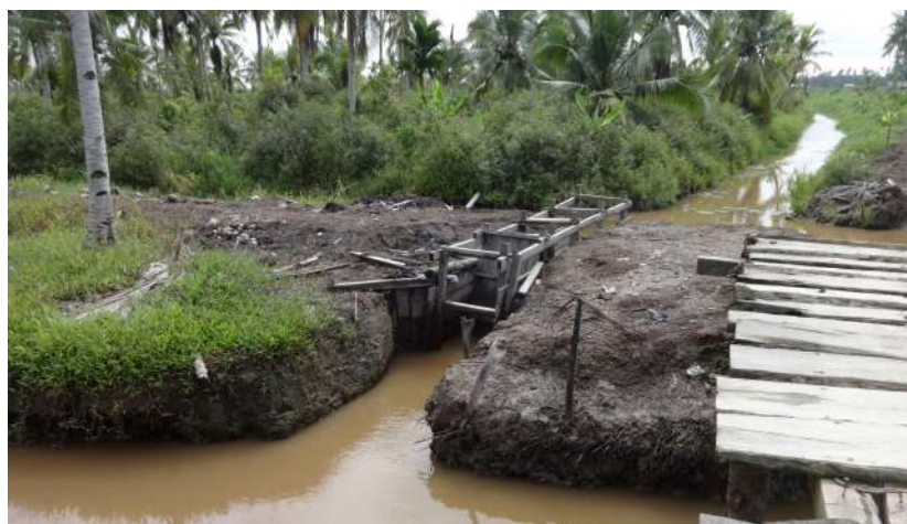
A Sluice Gate to Control the Flow Canal Water
